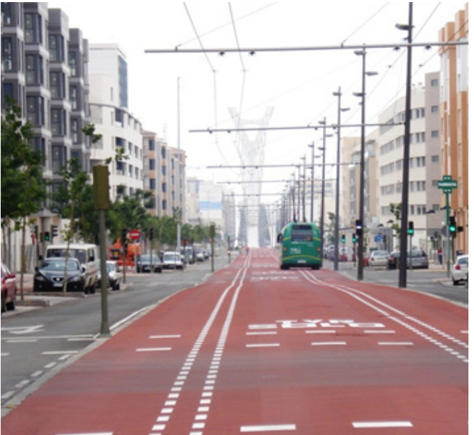
Example of a stretch of the dedicated lane segregated from the normal traffic
