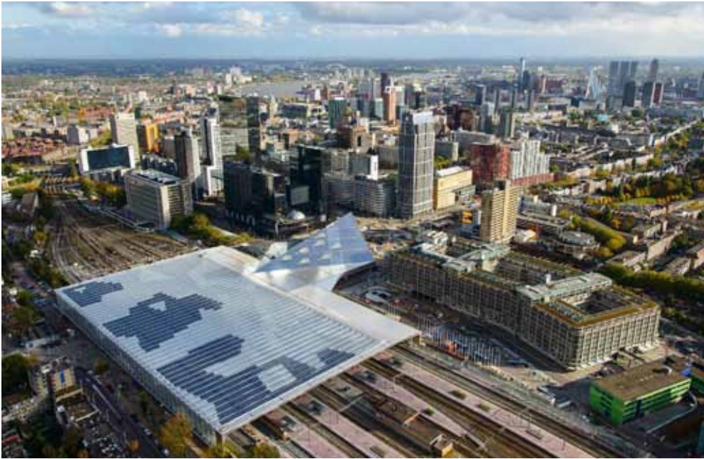
- Stationskap Station Rotterdam Centraal - verbindende factor-
